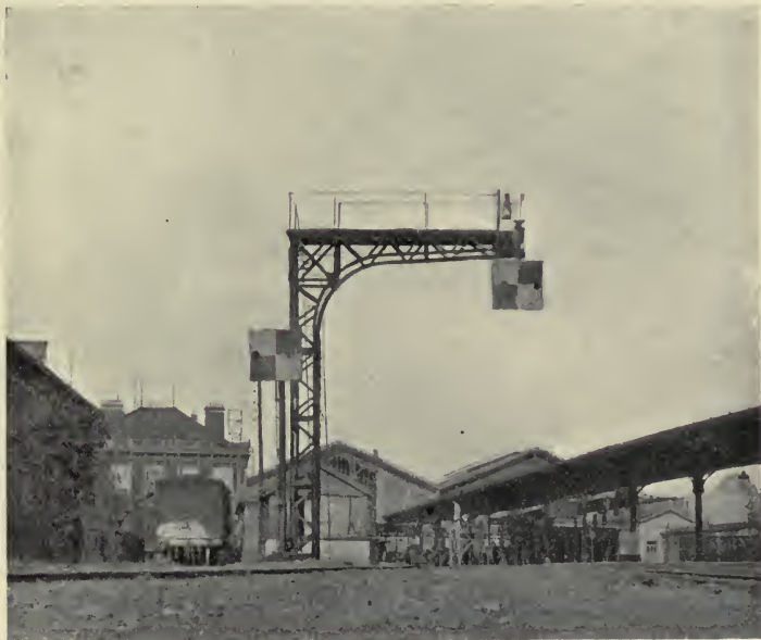
RED AND WHITE CHESSBOARD SIGNALS (NORD).
